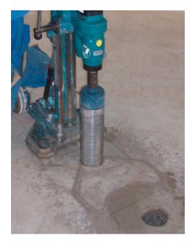
After marking the anchor holes, they will be drilled with a core drilling machine.
