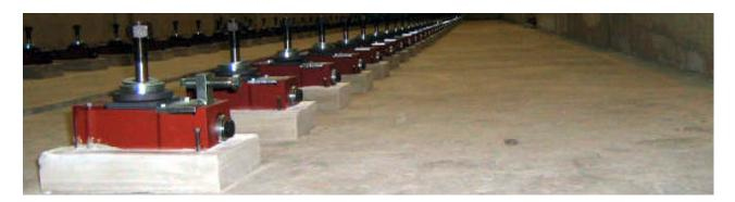
Positioned and grouted BW-Fixators®. Ready for machine arrival! 经过校准和灌封的固定器场地。机器可以登场了!
