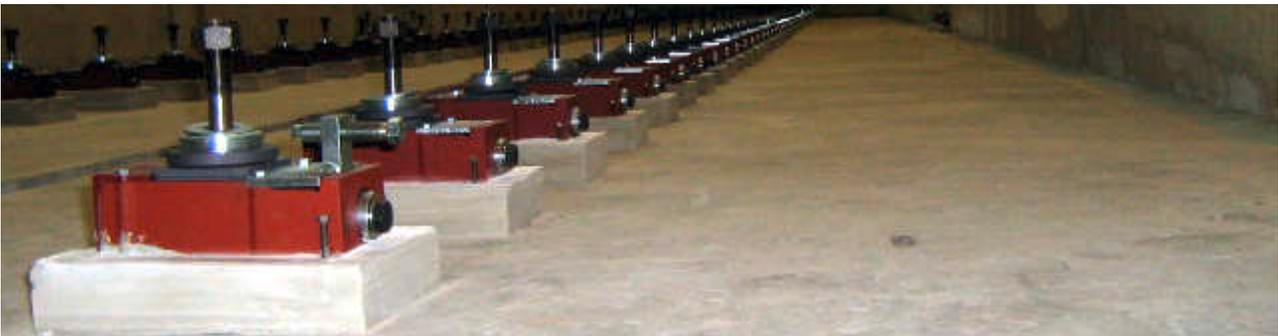
Positioned and grouted BW-Fixators®. Ready for machine arrival!
