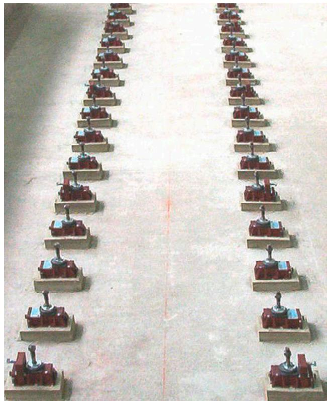
Grouting the BW-Fixators® and the anchor bolts will be done by our own engineers with non-shrink grout (Pagel V1).
