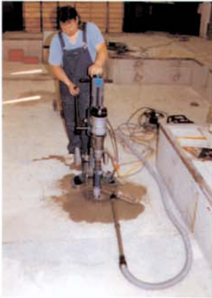
Drilling anchor holes with a core drilling machine
